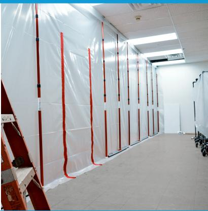
Armour Poly Sheeting Heavy rolls are a 2.1 mil thickness and used in many applications in construction such as temporary hoarding, dust control, restoration and abatement, and more.
