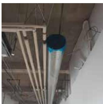
Armour Premium Duct Film provides reliable protection for uninstalled or partially installed ductwork, helping to maintain system cleanliness and integrity during construction or storage.
