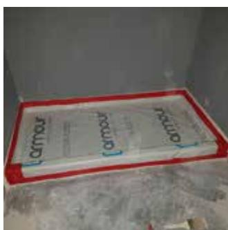
Armour Protection Fleece provides advanced temporary surface protection designed for curing floors and high-shine finishes, combining breathability, waterproofing, and durability for demanding jobsite conditions.
