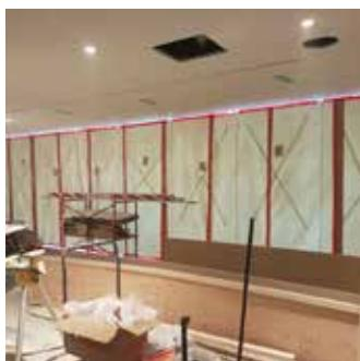
Armour Protection Paper provides reliable and economical protection for finished surfaces, making it an excellent choice for light-duty coverage during short project timelines in areas with minimal traffic.
