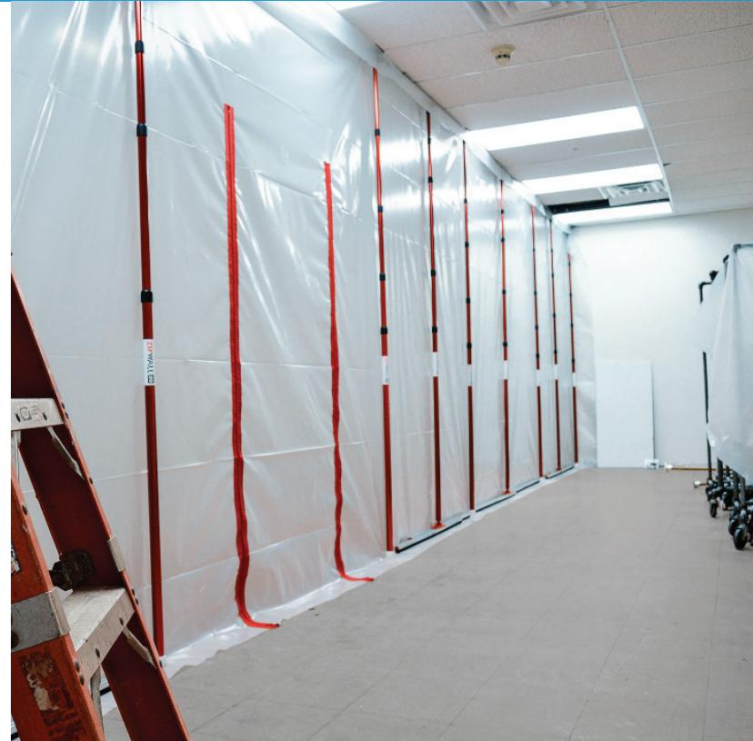
The Armour Poly Sheeting Roll - Heavy (Clear) is a versatile solution for temporary protection on construction projects, offering reliable coverage for dust control, overspray, and hoarding applications.
